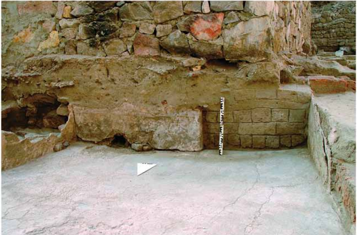
Fig. 12: Bathhouse. Southern wall with entrance and pipe for water-disposal
