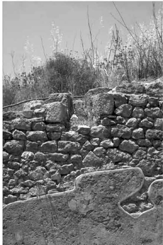
Fig. 2: Morgantina, House of the Doric Capital, Room 4, blocked window
