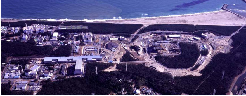
Figure 5: Photograph of the construction site taken in January, 2005.
