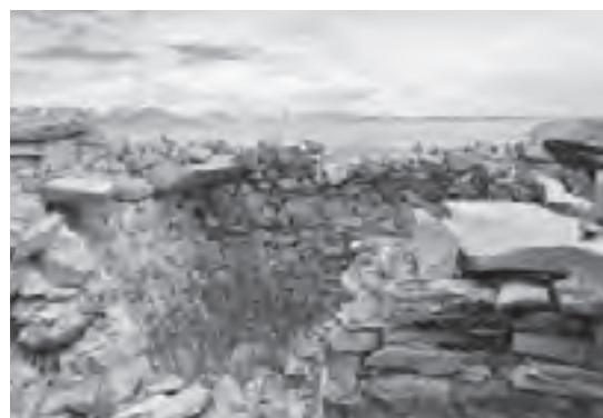
Fig. 73. Structure B3, Brag-sgam rdzong (B-40). Note corbelling protruding from the left wall
