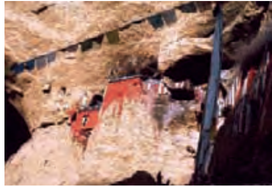
Fig. 110. The exterior of the Buddhist hermitage of Khwa-rtse . Note the wooden balconies and walkways extending out from the face of the complex
