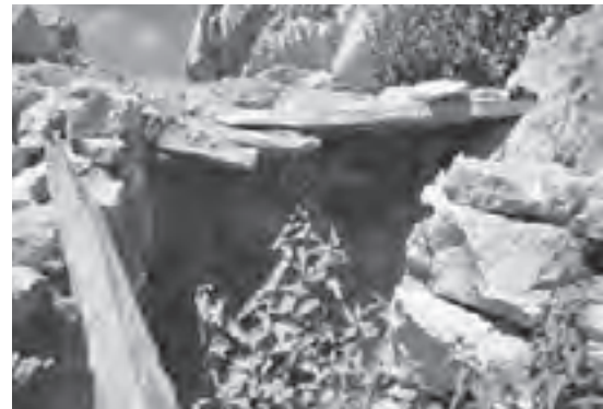
Fig. 98. The all-stone corbelled roof of a Dzong dkar-po (B-107) anteroom
