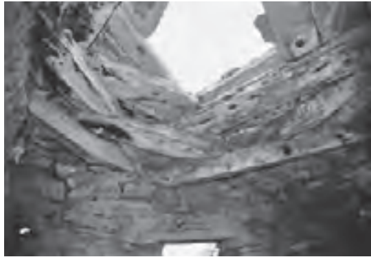
Fig. 1. A well-developed corbelling technique, gZims-phug (B-31)
