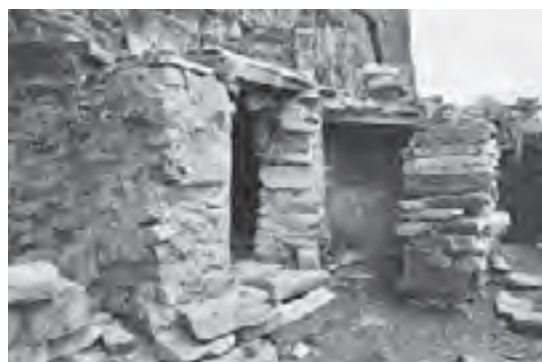
Fig. 87. A building with an all-stone corbelled roof, Shel-'dra (B-113). This cave hermitage was in regular use until the end of the pre-modern period
