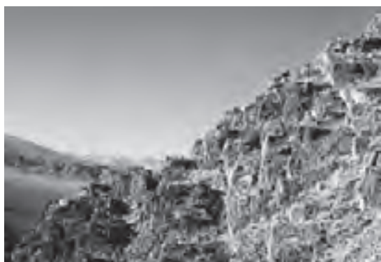
Fig. 52. The vestiges of an extensive network of defensive walls situated below the summit of the mKhar dkar citadel (A-109)
