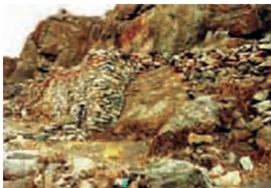
Fig. 102. The retaining wall at A-phug (B-115). This wall encloses a level area in front of the cave
