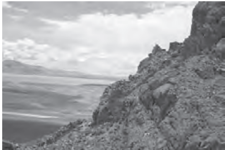
Fig. 57. The remains of a curtain wall and a vertical series of ramparts, Ser-mdzod rdzong (A-12). The southern portion of Dang-ra g.yu-mtsho spreads out in the distance
