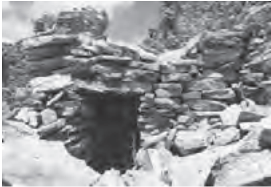
Fig. 9. An all-stone corbelled lower story underneath a superstructure that probably supported a wooden roof, dBang-phyug mgon-po mkhar (A-51)
