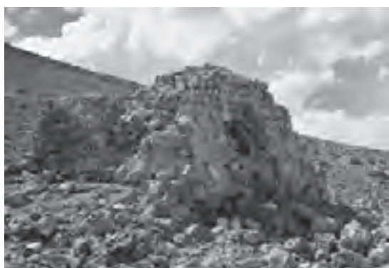
Fig. 237. Structure II (4 m x 7.8 m x 2.2 m), dPa'ngar gzhung khang-gog (F-1). This coursed-rubble structure has a very small interior cavity
