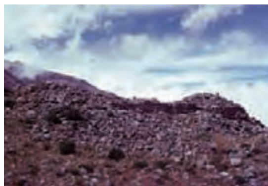
Fig. 141. An L-shaped temple-tomb, lower north complex, Yul kham-bu (C-143). The short side of the L-shaped structure (right side of the photograph) is 19 m in length while its long side is 55 m
