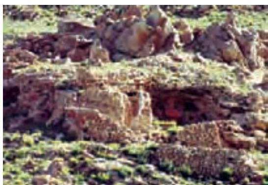
Fig. 103. The outlying walls of Lha-lung sgrub-phug (B-94)
