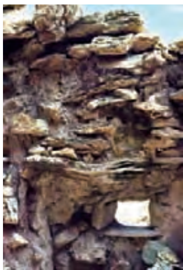
Fig. 99. A stone wall bonded with wood at the bTsag-tig (B-110) residential structure. The roof was also constructed using tamarisk ('om-bu) timbers
