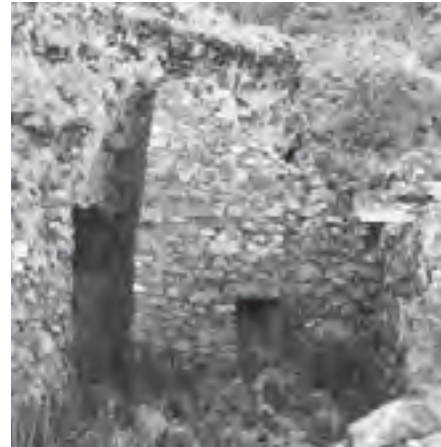
Fig. 94. The exterior wall of an anteroom, Am-nag (B-92)
