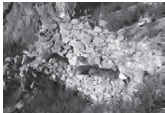
Fig. 4. Socketed corbels at the floor-ceiling juncture of what was originally a two-story structure, Phyug-tsho grog-po rdzong (B-6)
