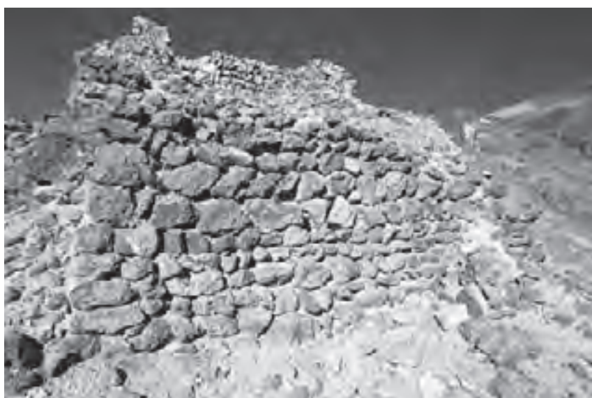
Fig. 245. Courses of stones placed horizontally and diagonally at the ruined citadel of mGar-gtsang mkhar (A-98)
