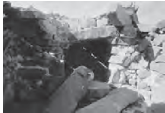
Fig. 2. An in situ corbel among those that have collapsed, mTsho-do (B-131)
