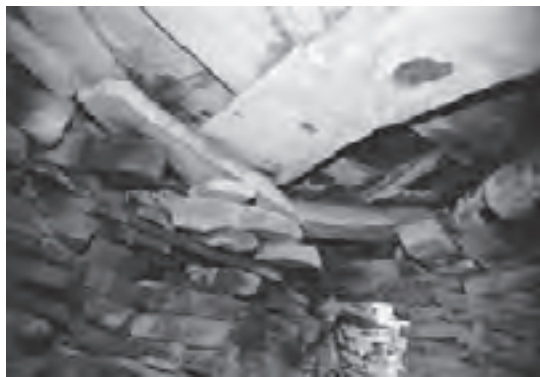
Fig. 3. Intact corbelling and bridging stones, Phug-chen (B-27)
