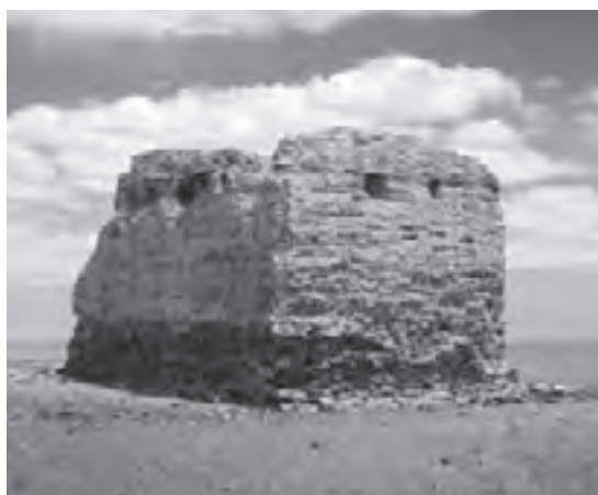
Fig. 70. Bu-mo lha-khang (B-87). This uniquely constructed edifice features a sandstone base, white earthen blocks and bluish seams
