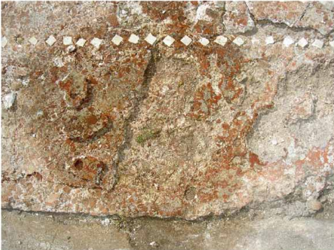
Fig. 10: Kalydon, House on the acropolis, detail
