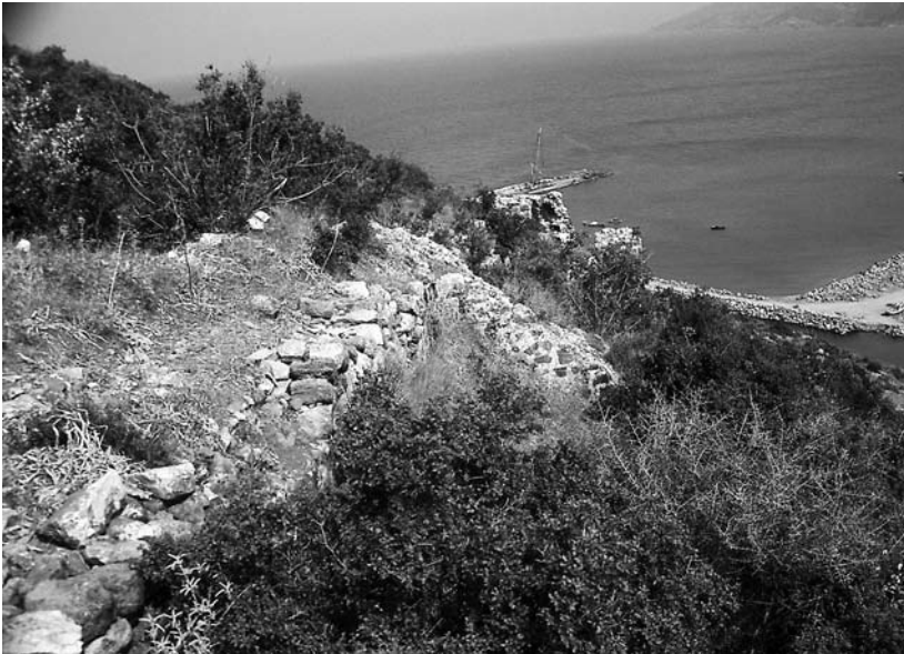
23 Circuit wall and tower, Selinus
