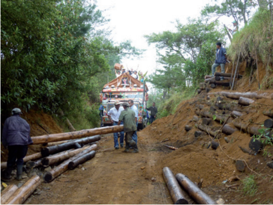
Figure 10 – Securing the roads.
