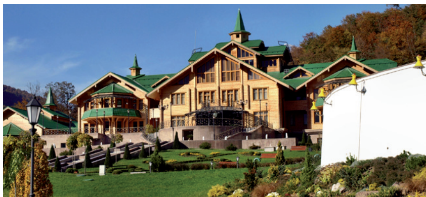
Figure 2 – Residence of the Russian President in Estosadok near Krasnaia Poliana. The (so far) only 5-star hotel in the valley and the ski lift of Gazprom are situated in close proximity. The lifts and infrastructure reach all the way to the boundary of the Kavkazki Zapovednik. © A. Borsdorf 2008
