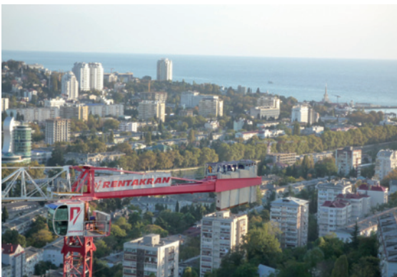
Figure 5 – The central district of Sochi. The political upgrading of the town through the regular visits by the president of the R.F. since the year 2000 triggered a building boom in the town. Lack of available land caused developers to build higher (background). The five-storey blocks of flats from the Chruschev era (mid-picture) are increasingly under pressure from newer buildings. © K. Scharr 2008
