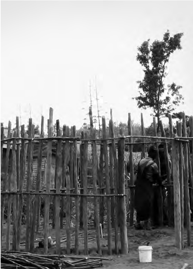
Fig. 9. Wall of vertical stakes under construction in Tanzania (Photo: Péter Timár).
