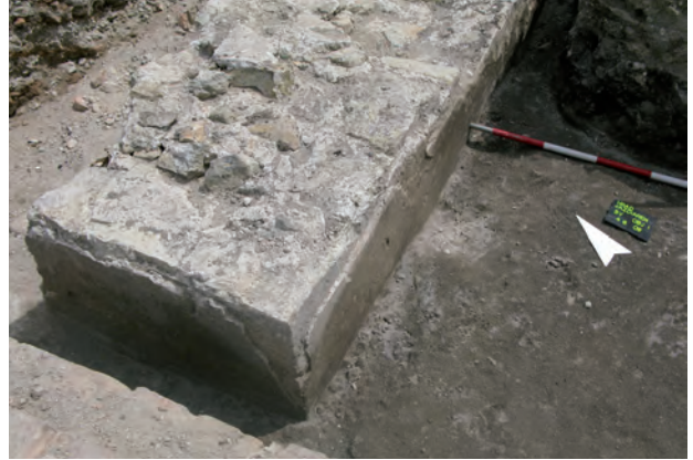
Fig. 6. Bratislava Castle – Winter riding school. The interior wall rendering of the corridor of the Roman Building I. View from the west (Photograph: M. Musilová; © MÚOP, Bratislava).
