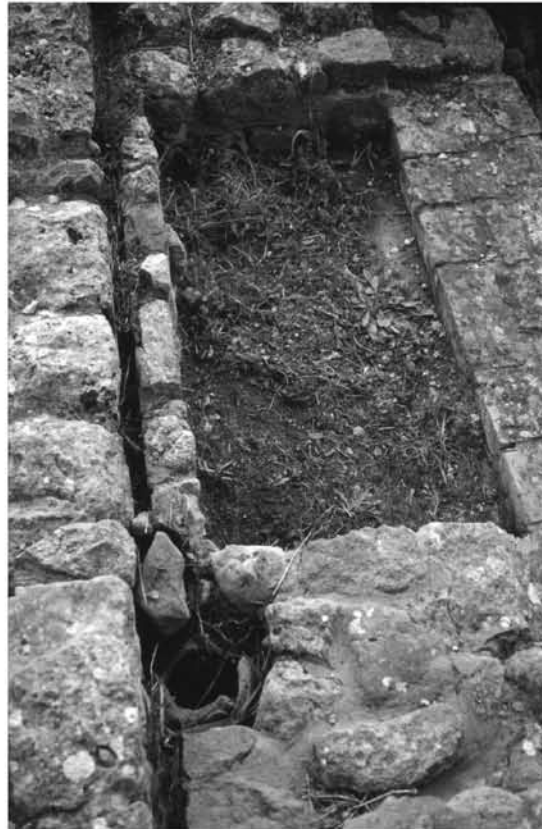
Fig. 15: Morgantina, House of the arched cistern, room 3: terracotta pipe (flue) in the southeast corner of the heated immersion bathtub; from southeast
