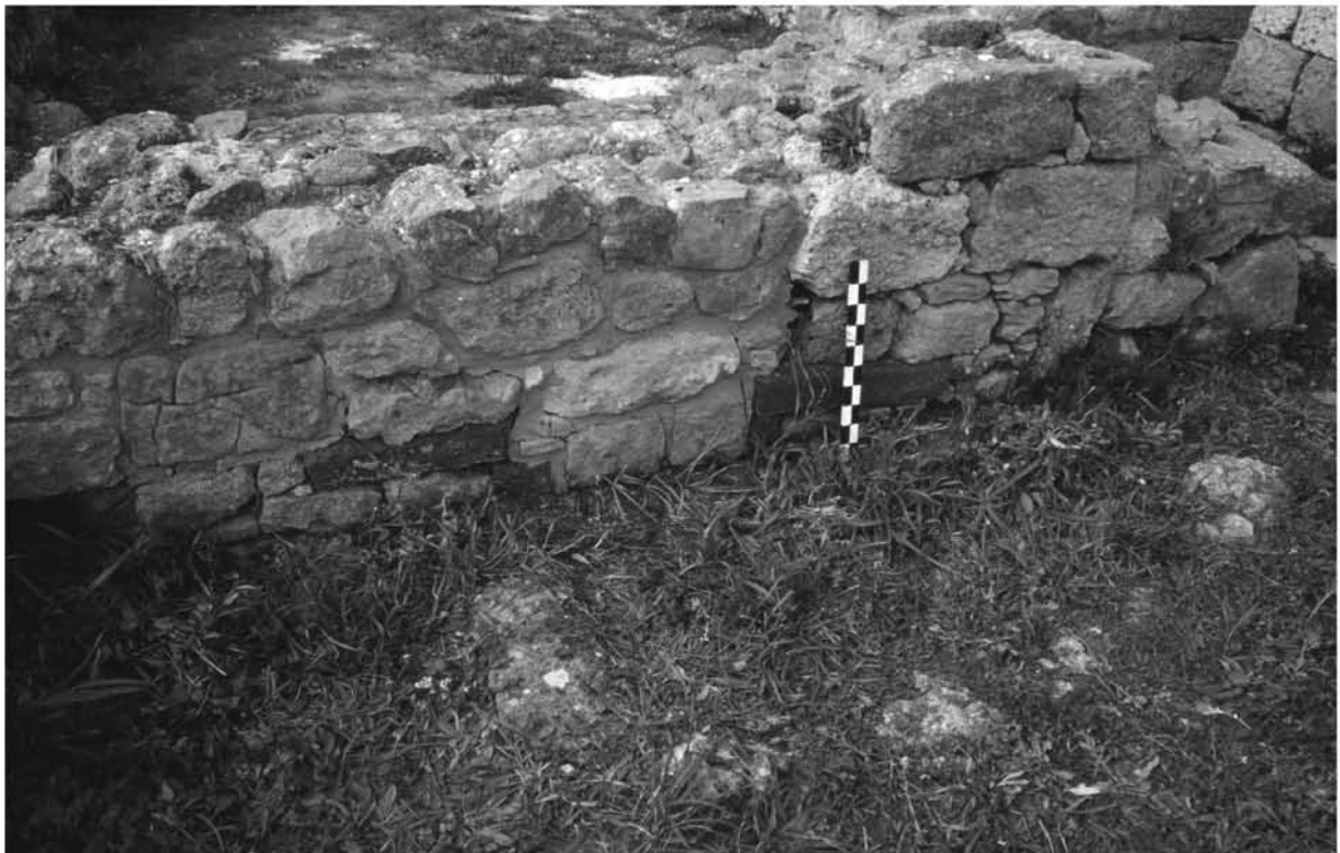
Fig. 14: Morgantina, House of the arched cistern, room 3: south wall of the heated immersion bathtub, blocked opening for heating the bathtub; from south
