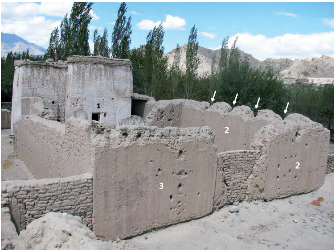
9. Assembly area of Temple 1 from south-east. Numbers indicate the walls numbers according to Fig. 8. The white arrows show the recesses where the beams used to fit on wall 2. The opposite wall has its top levelled (wall 3) (Q. Devers, 2009).
