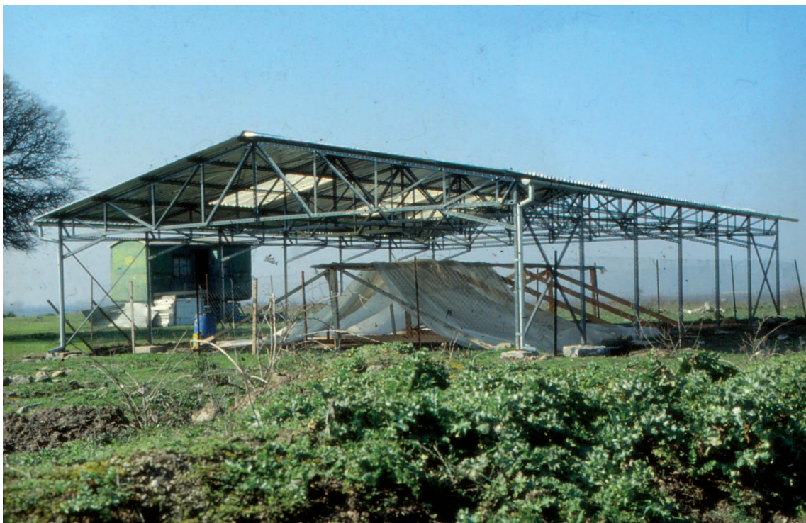
Fig. I.10 Metal pavilion above Trench A
