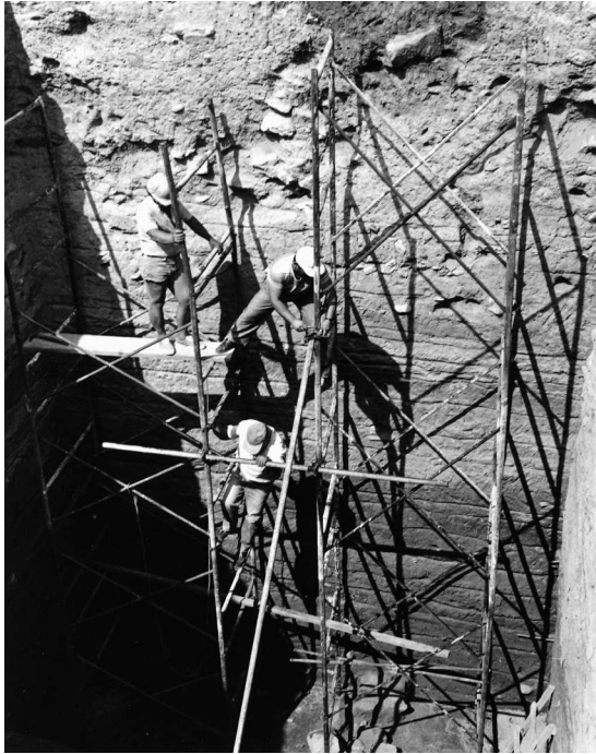
Fig. I.7 Constructing a metal scaffold to protect the sides of Trench A (09/08/1990)
