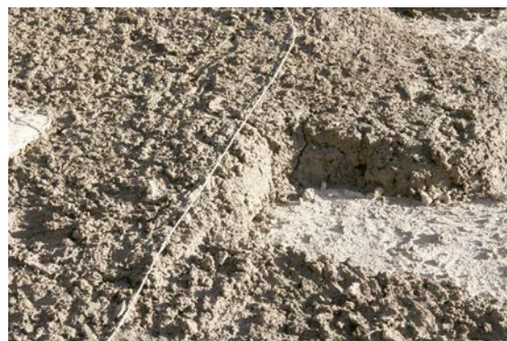
Fig. 3.24 (Right) Basgo. Maitreya Lhakhang. One layer of a mixture of thetsa and dzasa .
