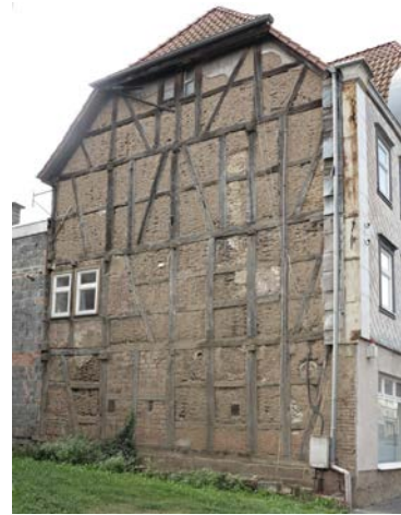
Fig. 4.5 Quedlinburg, Germany. Post and beam construction (c. mid 14 th century CE) filled with wattle and daub.
