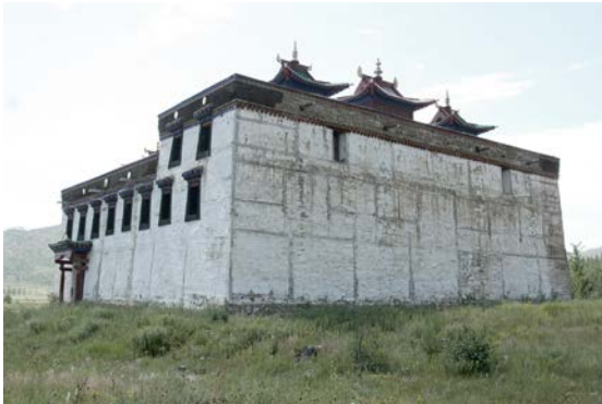
Fig. 4.9 Baldan Bereveen Khiid. Mongolia. Vertical and horizontal timber lacing in a solid wall.
