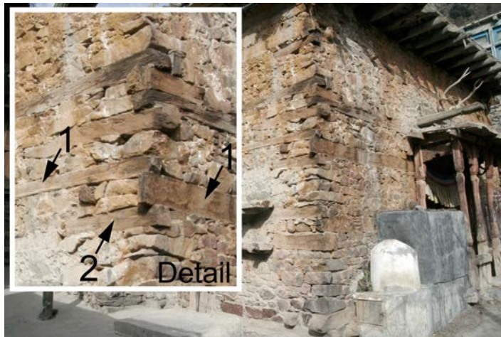
Fig. 4.66 Ropa. Lotsāba Lhakhang. South-east corner.
