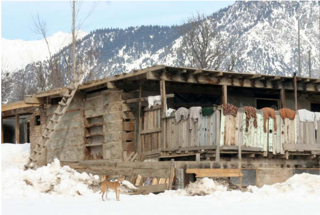
Fig. 4.48 Kalam, North Pakistan. Bhatar construction.
