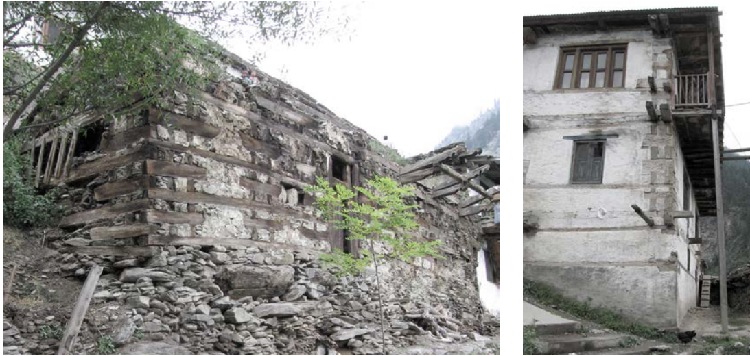
Fig. 4.96 (Left) Purthi, Chamba. Combination of dhol-maide and farque technique.
