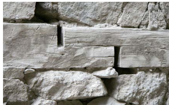
Fig. 4.32 (Left) Leh. Stone wall in the Old Town topped with an earth wall, both using timber lacing as crack stopper.
