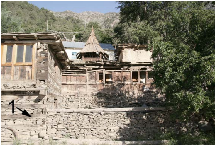
Fig. 4.74 Karla. In the picture left: kath-kuni construction (1).
