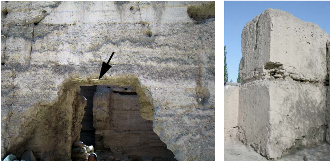
Fig. 4.30 (Left) Saspol. Ladakh. Rammed earth lintel of an entrance gate of the fortress reinforced with twigs.
