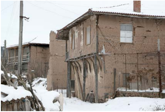
Fig. 4.16 Mandriza, Bulgaria. Adobe brick walls with timber lacing and a projecting upper floor.
