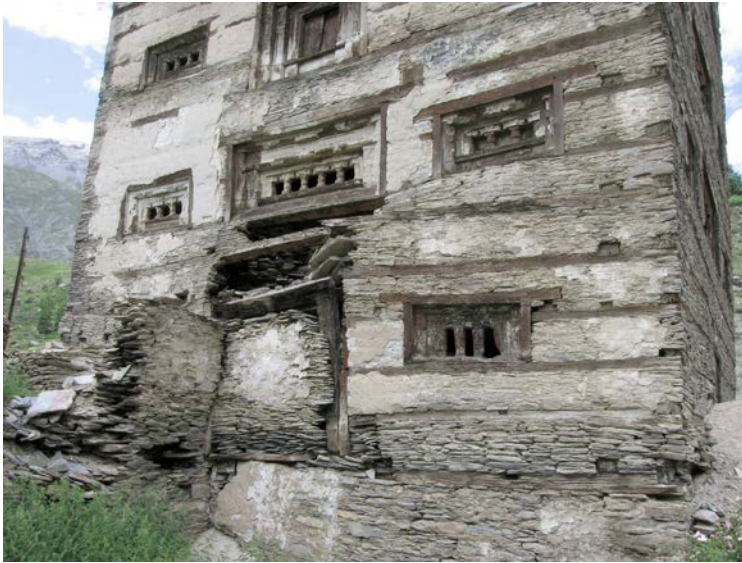
Fig. 4.21 Gondhla. Lahaul. Placing wooden window frames in a stone construction with 'ladder'-like timber lacing.
