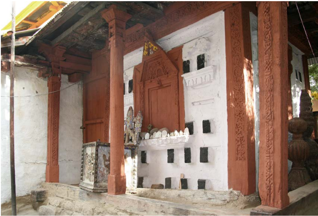
Fig. 4.91 Ribba. Middle Kinnaur. North facade.
