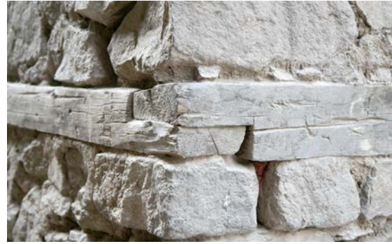
Fig. 4.33 (Top) Leh. Old Town. Corner half lap joint.
