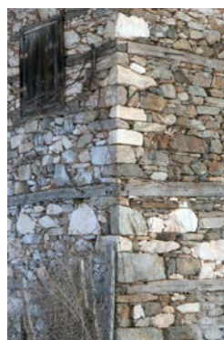
Fig. 4.19 Dolno Lukovo. Corner half lap joints.
