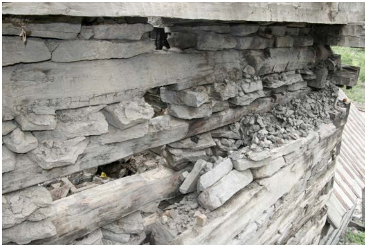
Fig. 4.89 Kalpa. Interior of the kath-kuni wall between the runner beams is filled with rubble stone.
