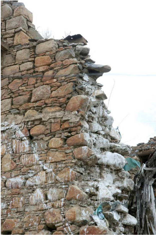
Fig. 4.14 Lhasa. Tibet. Traditional technique of stone laying shown at the Shide Lhakhang.
