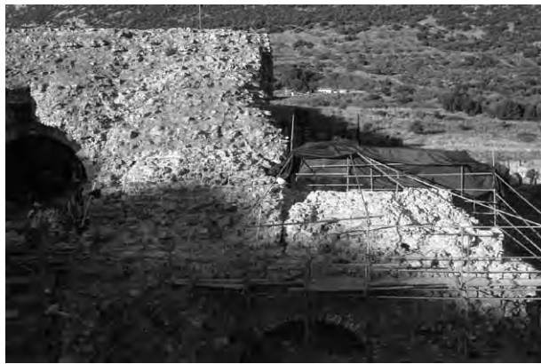
40 View of the area above the S1 vault after the cement-based capping was stripped
