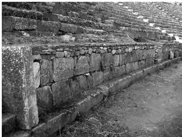
24 Portion of the second diazoma wall before consolidation
