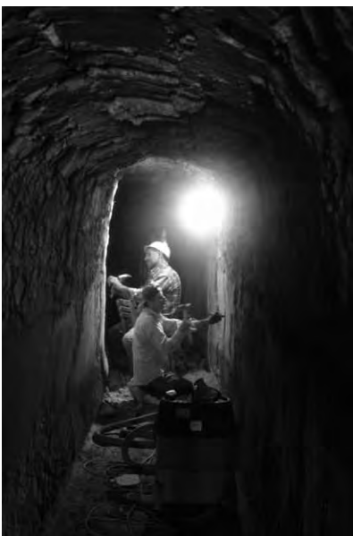
45 Consolidation work in the water channel below the substructure chambers of south analemma
