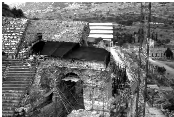
41 South analemma during the course of interventions
