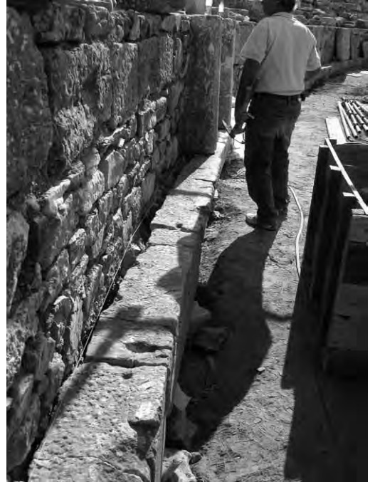
30 Process of placing the pedestal blocks back in their positions
