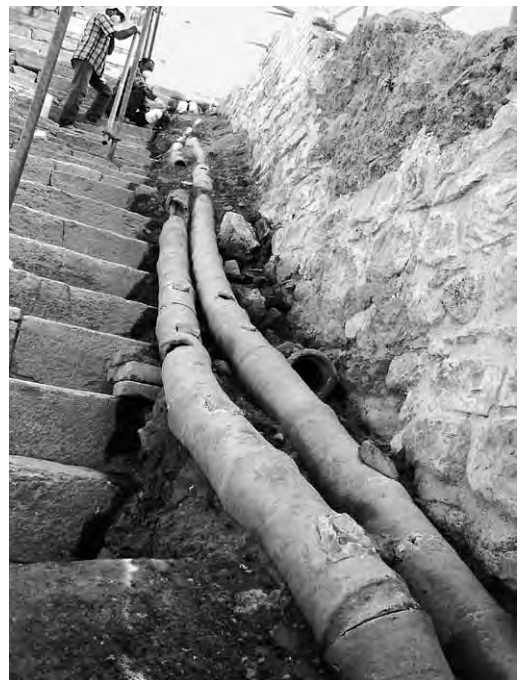
33 Consolidation of the mortar of the water pipes with ethyl silicates
