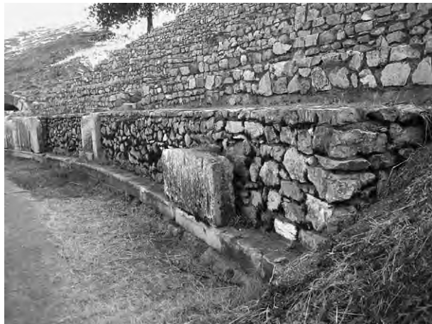
23 Portion of the second diazoma wall before consolidation
