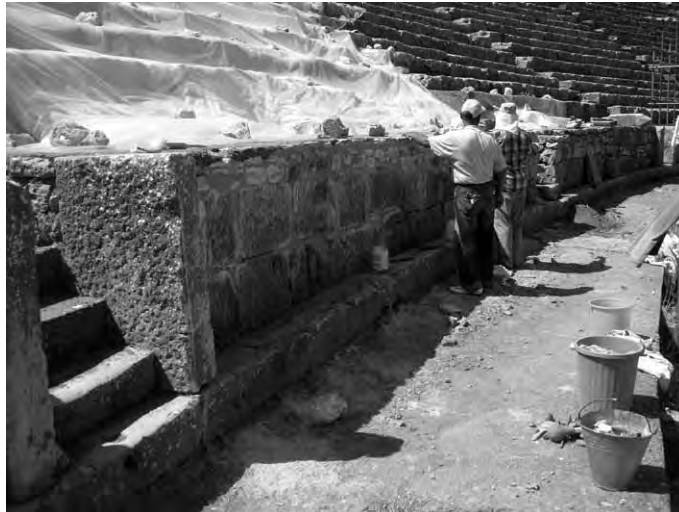
26 Second diazoma wall, after consolidation
