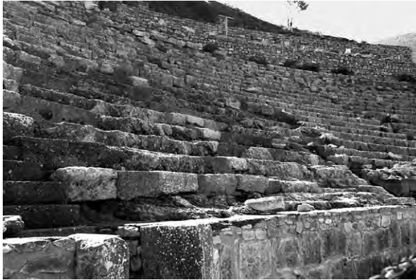
35 Conglomerate bedrock in summa cavea after cleaning and consolidation
