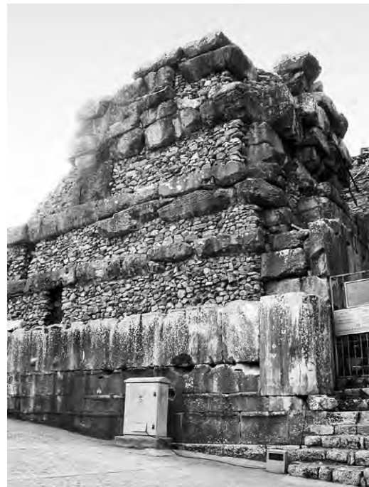
8 Structural reinforcement of wall core using rubble stone and cement based mortars at the south analemma
