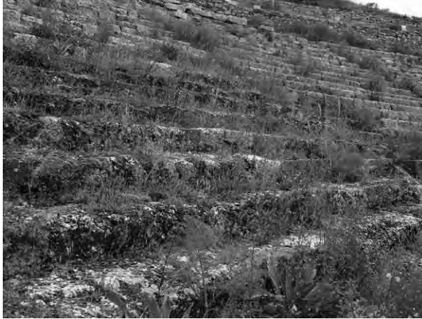
34 Conglomerate bedrock in summa cavea before consolidation
