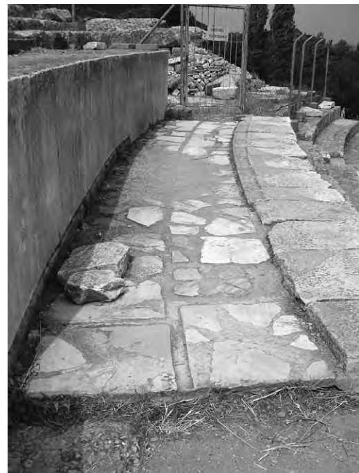
4 Reconstructed portion of the south end of the first diazoma
