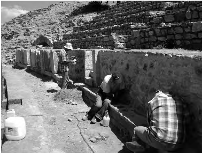
25 Second diazoma wall, after consolidation
