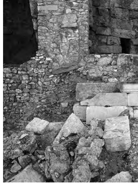
44 Rubble mass at the foundation of adjoining wall of south and north substructure chambers
