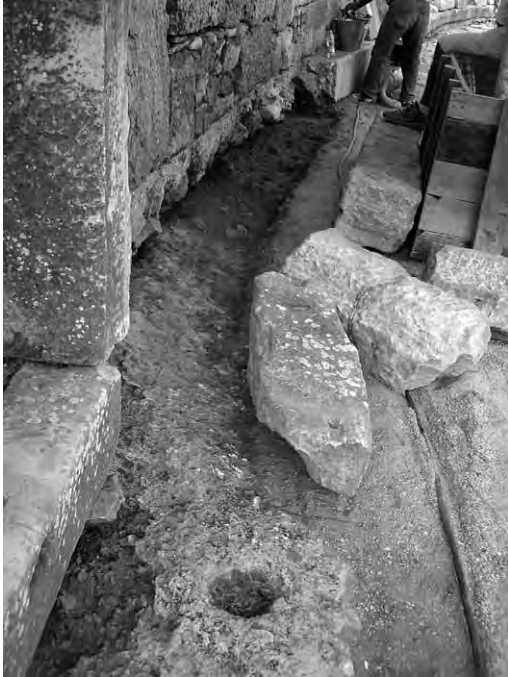
29 Excavated area in front of the second diazoma wall revealing a foundation of conglomerate bedrock
