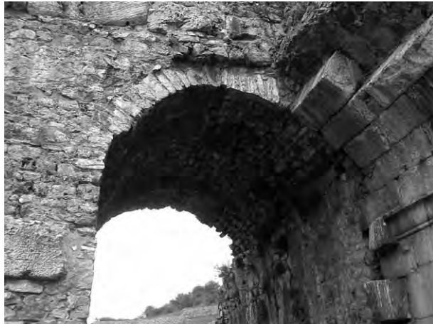
39 Interior of S1 vault prior to work seen from the south
