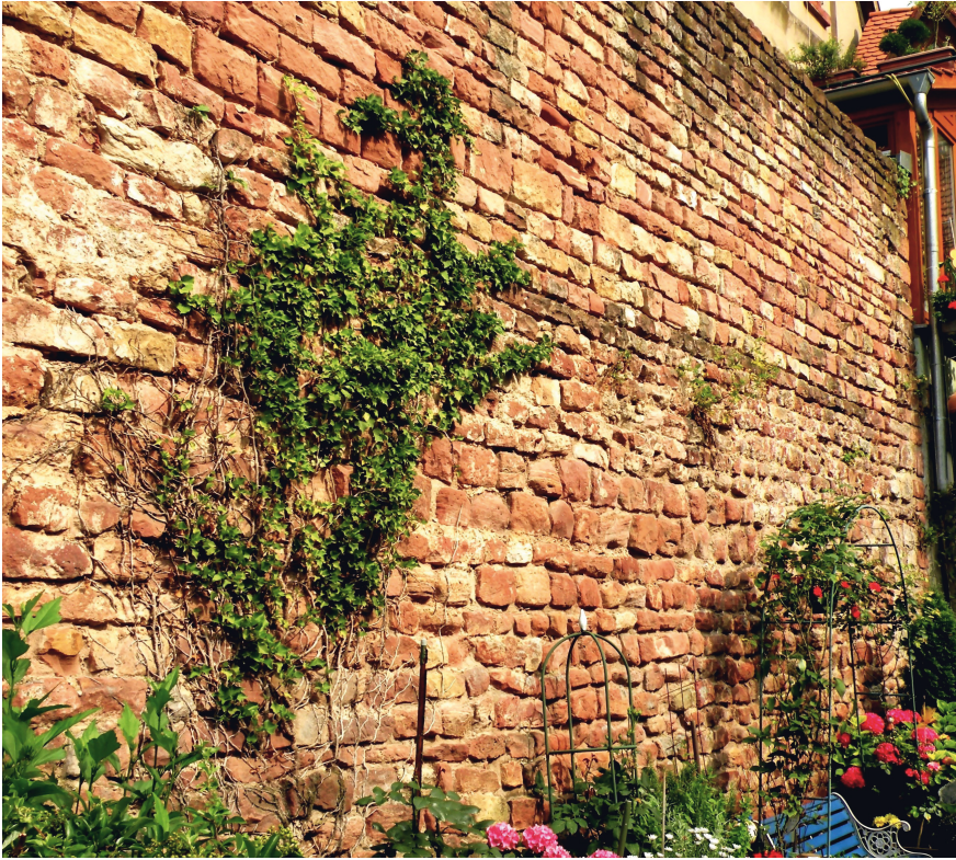
Fig. 3. A surviving wall of the fort built in Alamannia at Lopodunum (Ladenburg) by Julian and then expanded ca. 370 by Valentinian I, probably with the assistance of the Alamanni (Photo: author)
