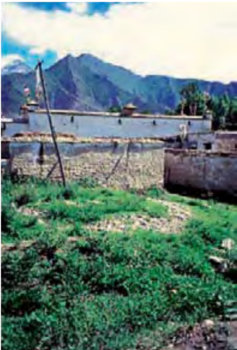
36. The pile of stones are the last remains of the khri dpon palace in Tshal. It is also locally described as the “birth place” of the protector god Pehar (2001)
