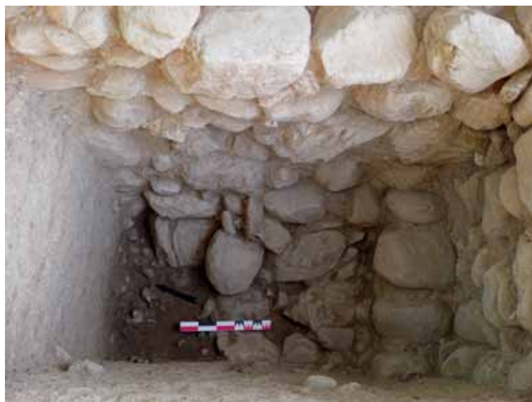
Fig. 7: Building Δ. The foundation of Walls 104 (top) and 102 (right) (photo copyright: A. Vasilogamvrou)
