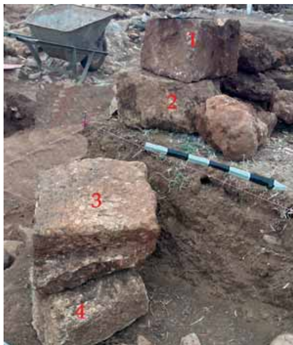
Fig. 6: Ashlar blocks from the Cyclopean Terrace Building
