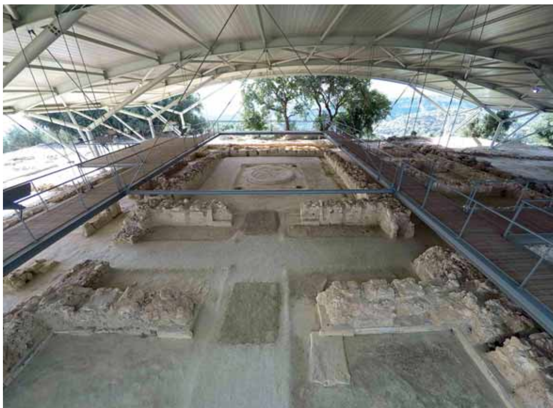
Fig. 2: New shelter over the central corridor of the Palace of Nestor, June 2016, looking northwest (Ephorate of Antiquities of Messenia/Department of Classics, University of Cincinnati)
