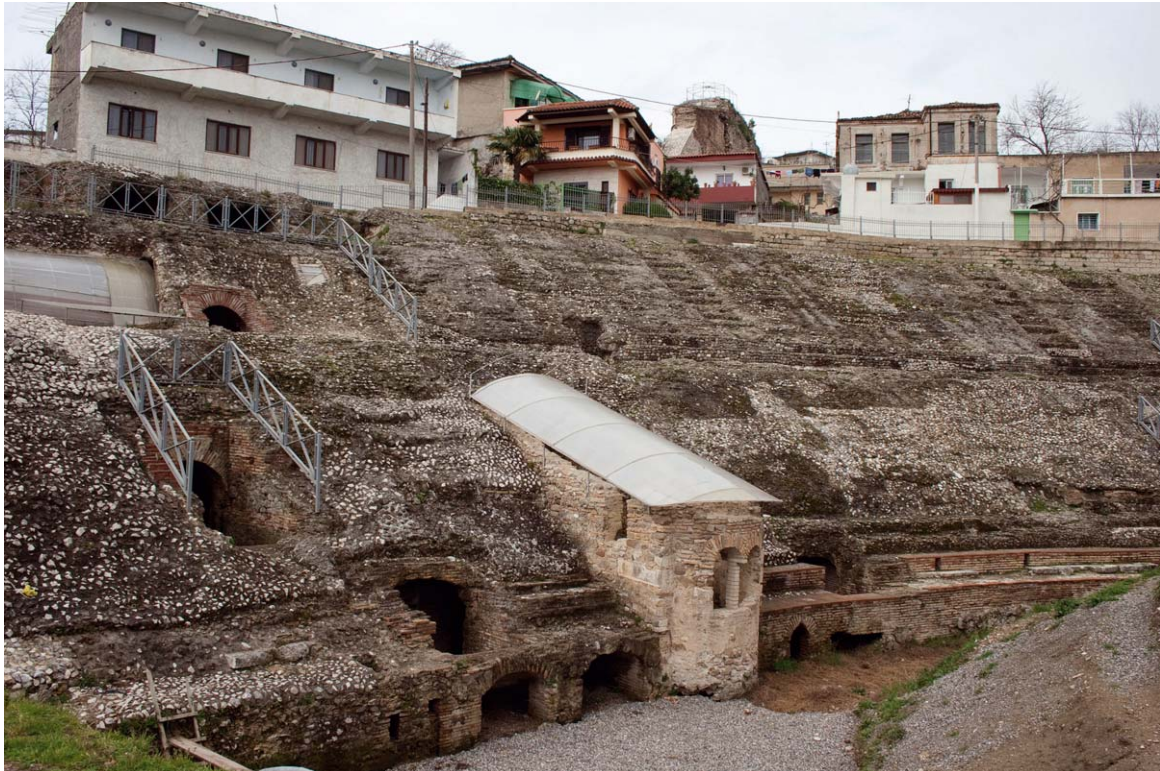
Fig. 1: Amphitheater of Durrës, view of the chapel from the southeast (Photo: G. Fingarova).
